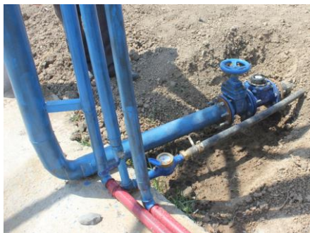
Valve and water meter:
