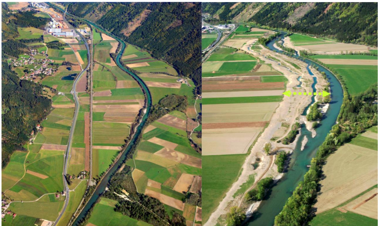
Fig. 15: Detail of river bed enlargement on the same site.
