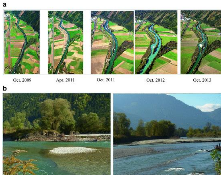
Fig. 14: One of the sites of intervention along the Drava River.
