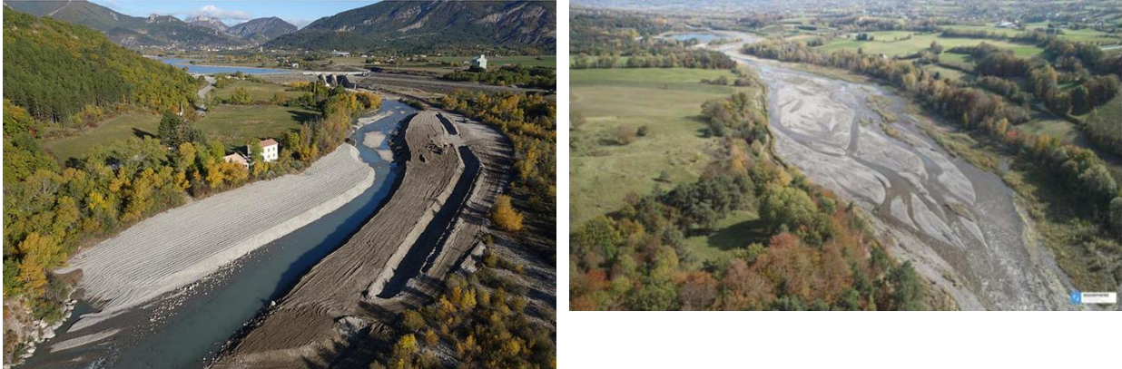
Fig. 13: Left: artificial gravel replenishment downstream from Saint-Sauveur dam. Right: aerial view of the restored reach of the Upper Drau in 2018, showing the spontaneous recovery of the braided channel.
